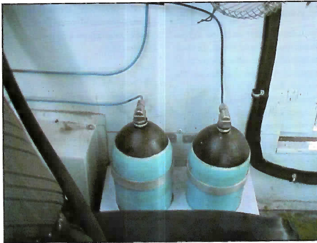
Fig-2: Oxygen cylinders
