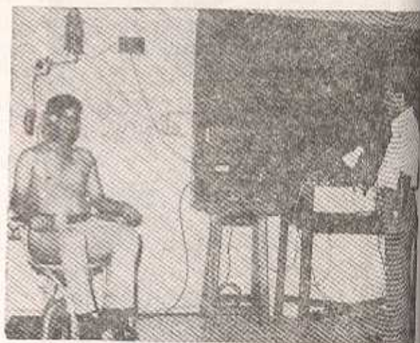
Fig. 4 The test set up with Barany Rotation Chair, Control panel and Electro-stagnograph. Subject being rotated with head in central position
